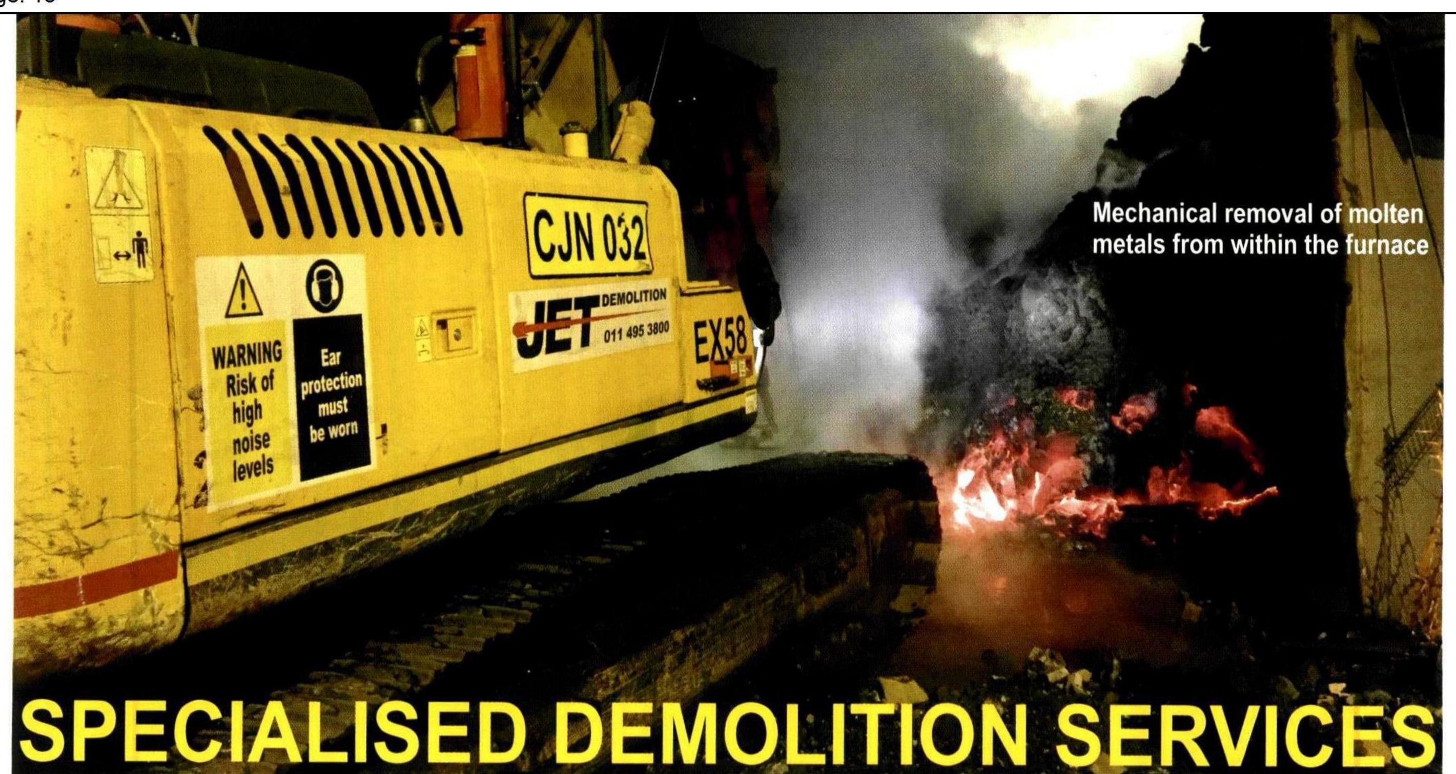
Furnaces in the steelmaking, glass, or general transition seamlessly from stave-jacking to lancing and to
